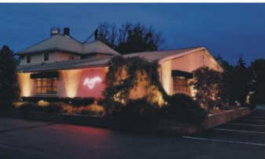
Using just three types of lights, the job dramatically highlights the restaurant's walls and landscaped areas. The effect is colorful, but the bright tones are derived exclusively from the neon sign and wall paint.
